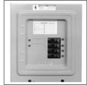
Know the location of the circuit breaker panel. Label the breaker that controls your kiln's circuit.
