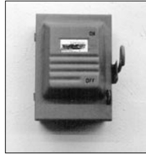
Be sure the power disconnect switch is in the on position.
