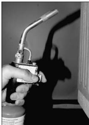
After you have cemented the brick patch, heat the cement seam with a propane torch. Hold the torch 5 - 6 inches away from the firebrick surface for about 10 seconds. **Move the torch back and forth so the firebrick does not get too hot in one place.** (Otherwise you may heat-shock the wet cement.) Let the patch dry overnight before firing the kiln.
