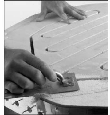
If you are coating over a freshly patched firebrick surface, allow the cemented patch to dry first.
